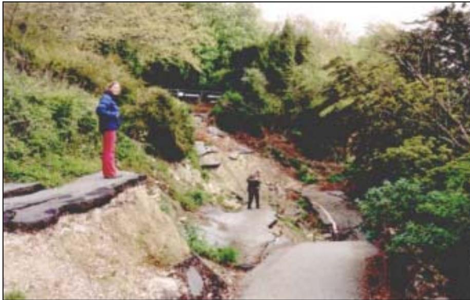
*Fig. 9: Severe damage to the A3055 as a result of coastal erosion and ground instability.*
