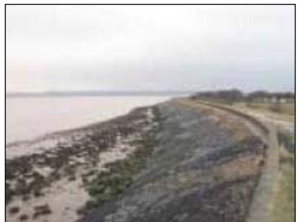
Fig. 13: Stone protection in Humber estuary.
