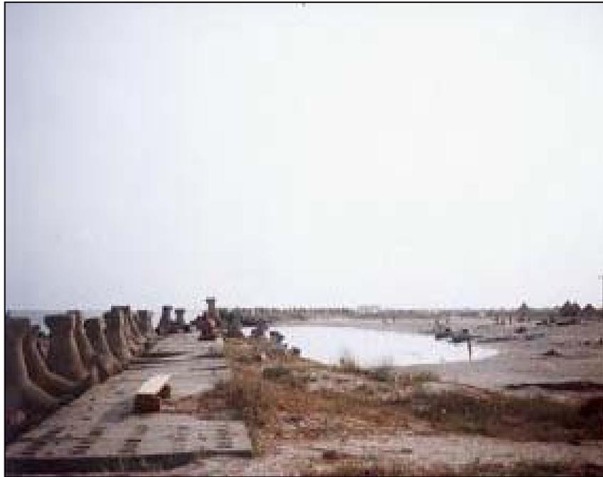
*Fig. 9: Protection dyke using tetrapods and concrete platforms (Portita beach).*
