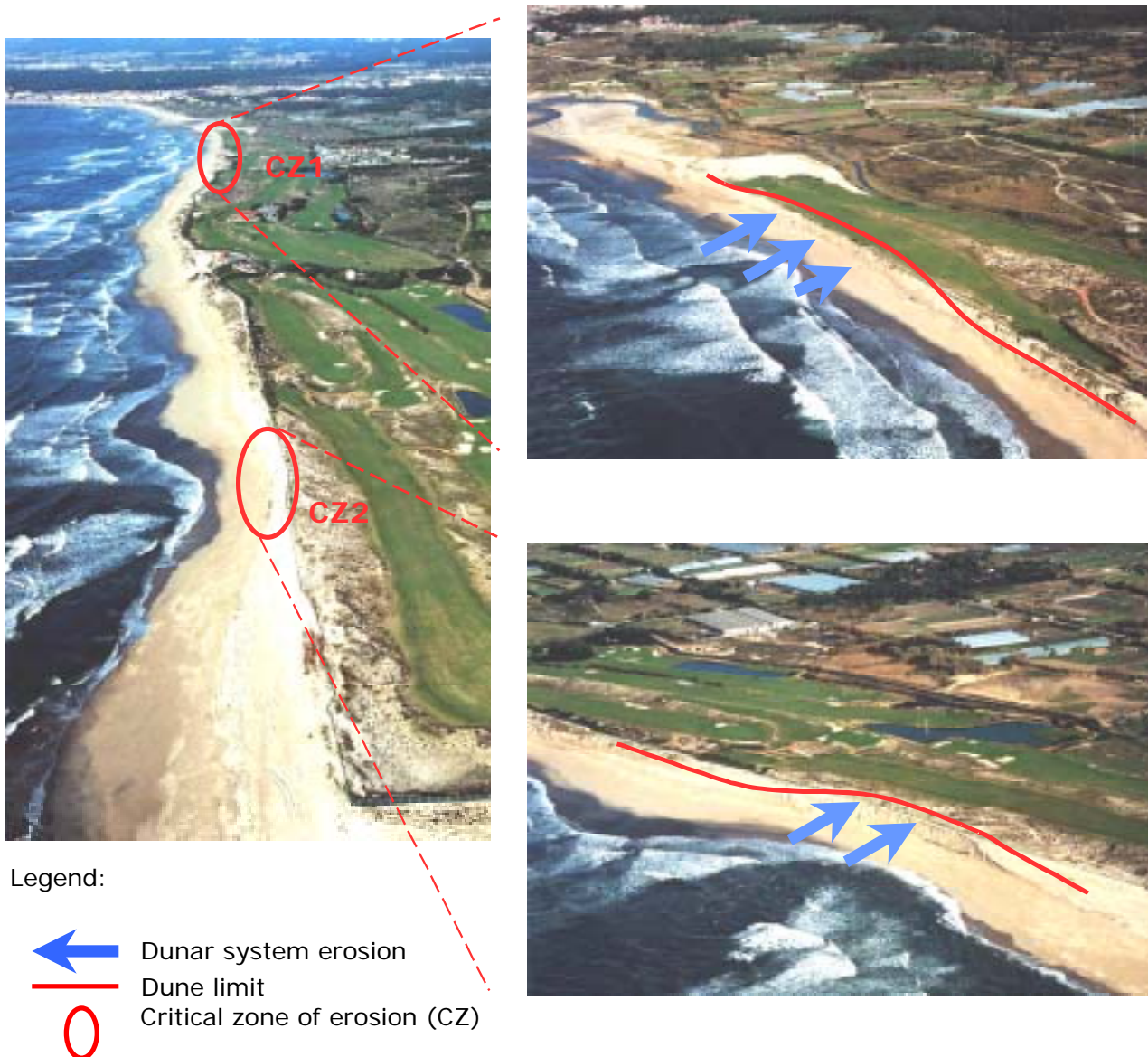
Fig. 8: Estela golf course, critical erosion zones (Aerial photographs: F. Piqueiro, 1997).
