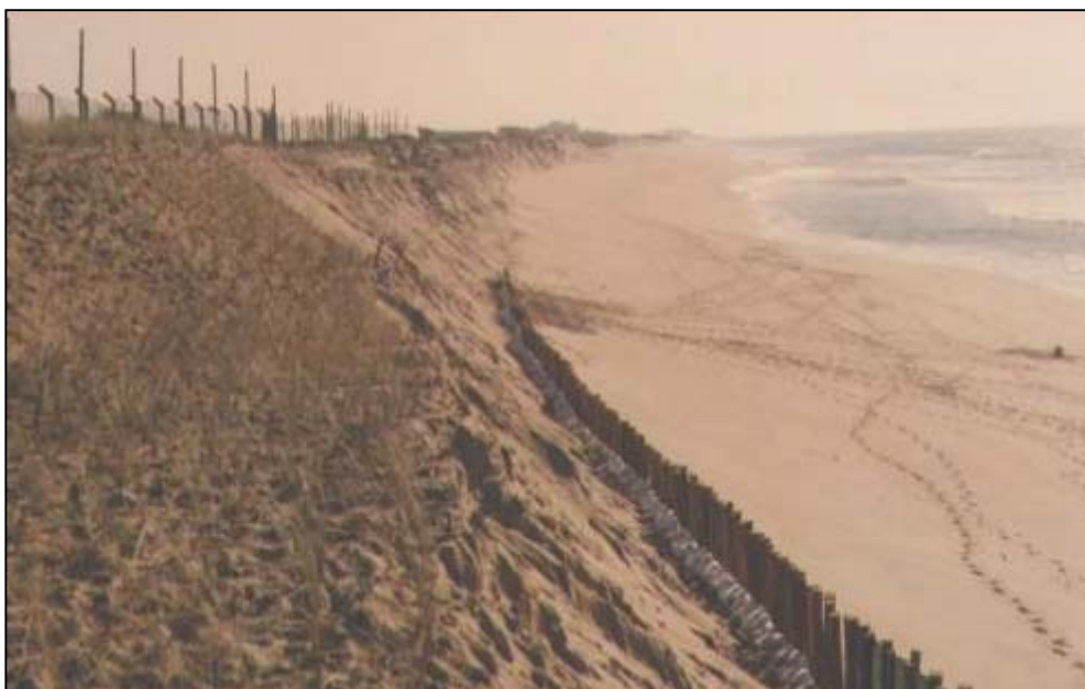
Fig. 9: Dune consolidation with wood piles and small sand bags, April 1999.
