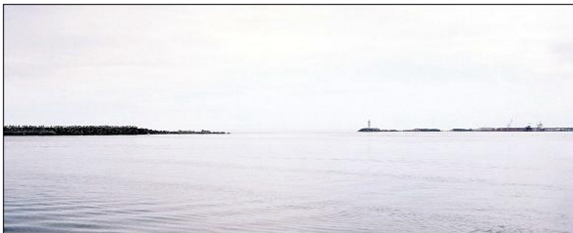
Fig. 22: “Praia da Vitória” harbour entrance, after the destruction provoked by the storm of December 2001.
