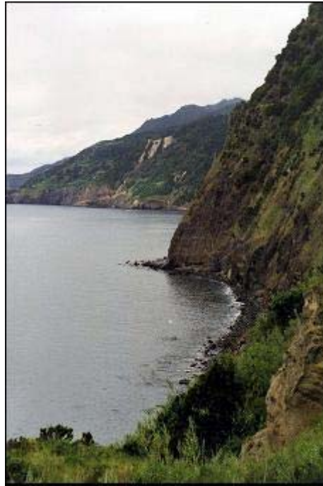
Fig. 5: Eroding cliffs on the São Miguel coast zone (F. Taveira Pinto, 2002).
