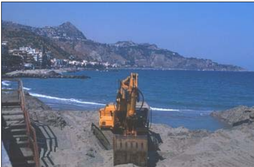
Fig. 10: Renourishment works in San Giovanni.
