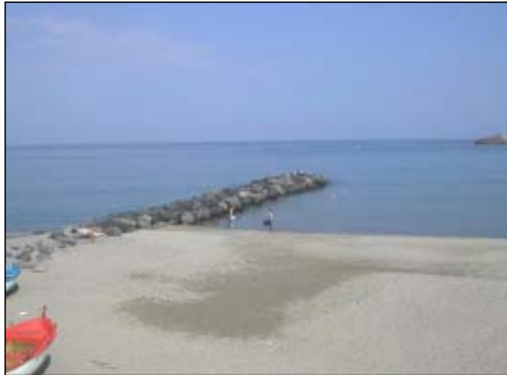
Fig. 7: Groyne structure in San Pancrazio.
