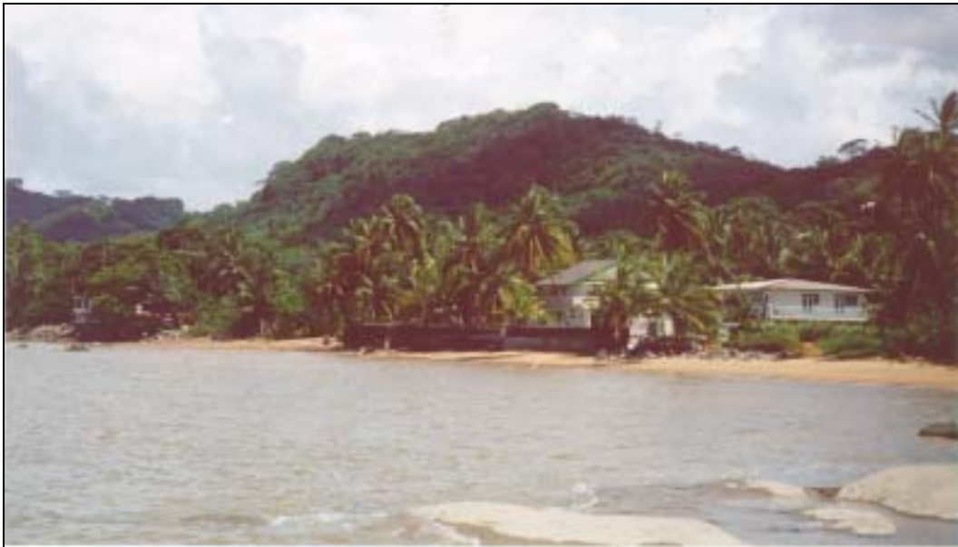
Fig. 5: Erosion of the north part of Anse de Rémire.
